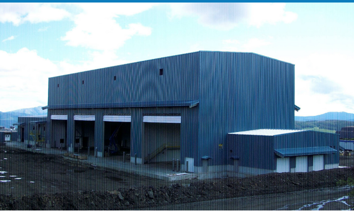
MINE BRULE - WESTERN COAL
